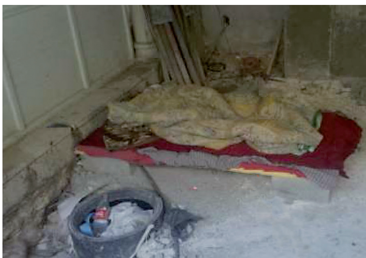
The illegal building from 2011 has been used since the summer as a lodging for illegals.
